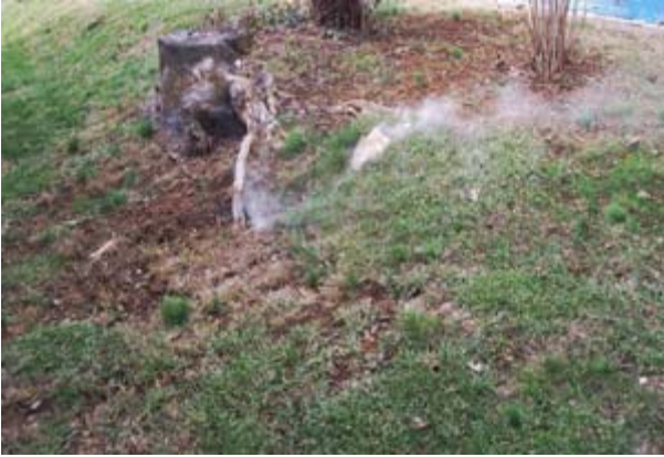
Smoke exiting ground
