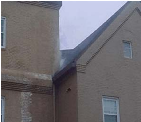
Roof drain connected to sewer
